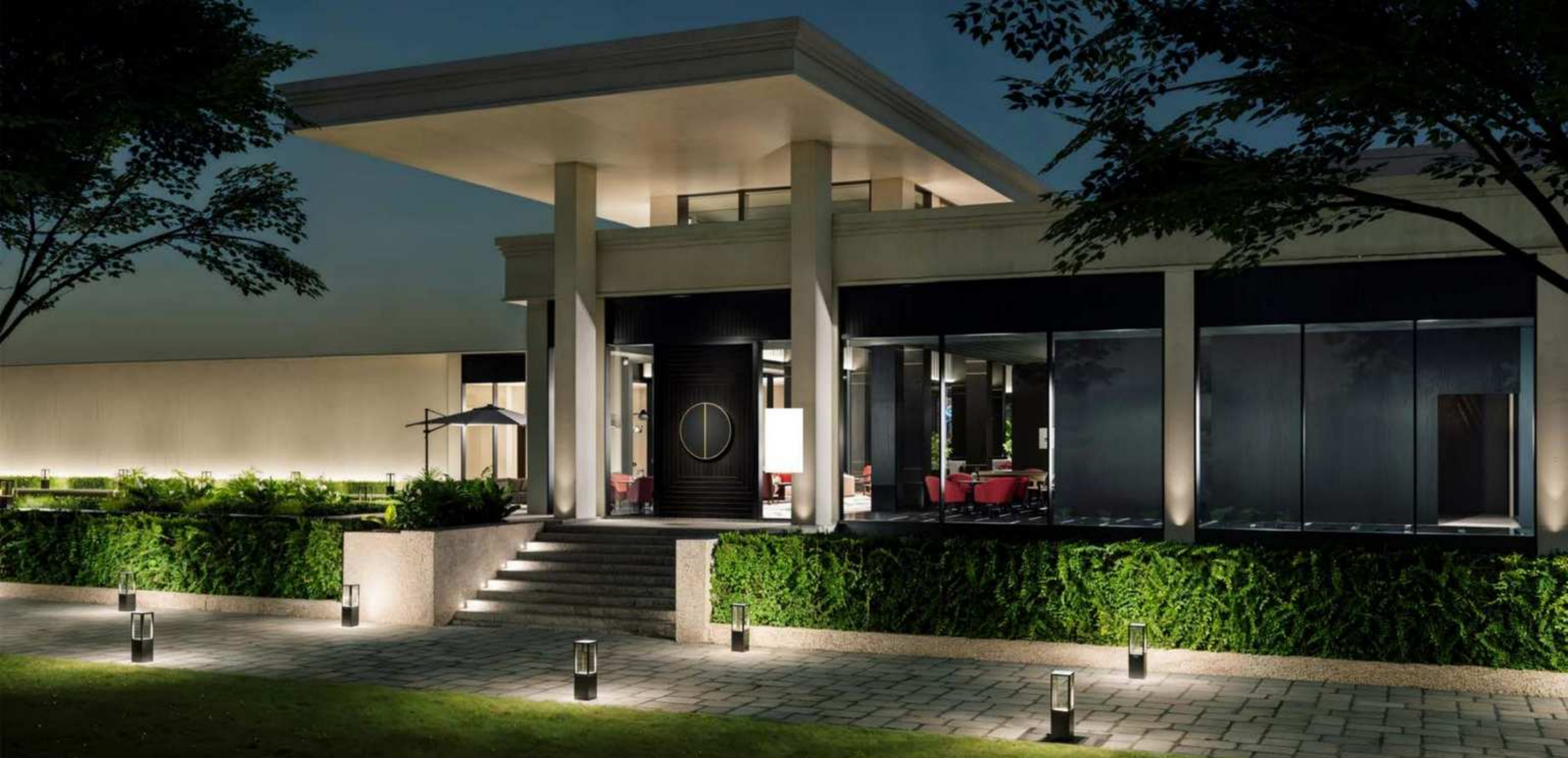
CLUB - Night Facade
